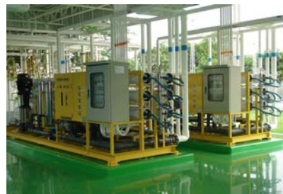
Recycle system of Treated water
