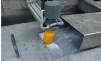
Drain gutter (over flow)
