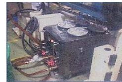
oil filtration (to filter contamination from oil)
